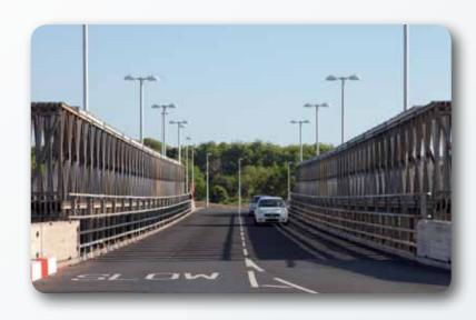
Janson's Panel Bridge system (code JPB) is designed for temporary and permanent applications wherever bridges with spans up to 400ft (122 meters) for all general traffic are required. The system is based on the original Bailey Bridge concept using trusses assembled from modular panels.
