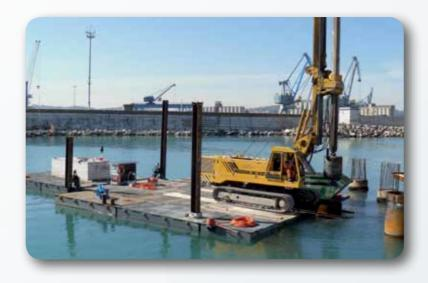
Janson's modular Couple Pontoons (code JCP) assure a quick, easy and inexpensive way to create platforms on water. They are used for civil works enabling cranes, excavators or drilling machines to work on water, for landing stages and for special events such as stands, theatre sets, firework shows etc.
