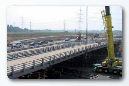
Janson's Plate Girder Bridge units (code JSB) are designed for temporary and permanent applications particularly in areas of heavy traffic conditions where single spans up to 40 meters for all general traffic are required.
