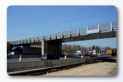
Janson's Beam Bridge units (code JSK) are designed for temporary and permanent applications wherever short span bridges up to 21 meter for all general traffic are required.
