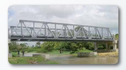
Janson's Truss Bridge system (code PSB) is a permanent structure that has been particularly developed for rural areas infrastructure where resources and transport facilities are limited, for emergencies (floods, earthquakes) and for peace keeping operations.
