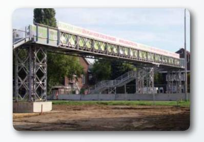
Janson's modular Pedestrian Bridge range consists of two systems: the Janson Pedestrian Panel Bridge system and the Janson Pedestrian Truss Bridge system.
